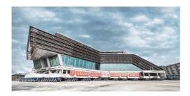
The modularity and combinability of SCHEUERLE SPMT axle lines allow the number of axle lines to be flexibly adapted to the respective payload requirement. This enables customers to successfully undertake spectacular projects. Shown in the photo: a 7,500-tonne hotel in China was moved 500 metres on SCHEUERLE SPMT due to environmental protection requirements.
